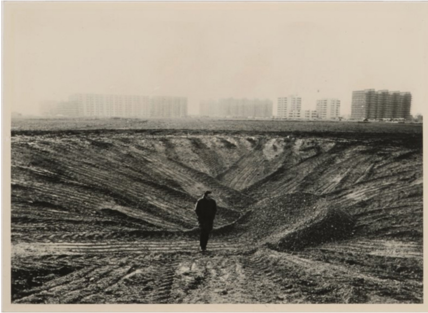
Imagen 9. Michael Heizer, Munich Depression, 1969. (Final stage), Munich.
